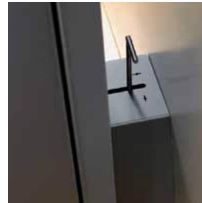
Shield and damper behind stove
